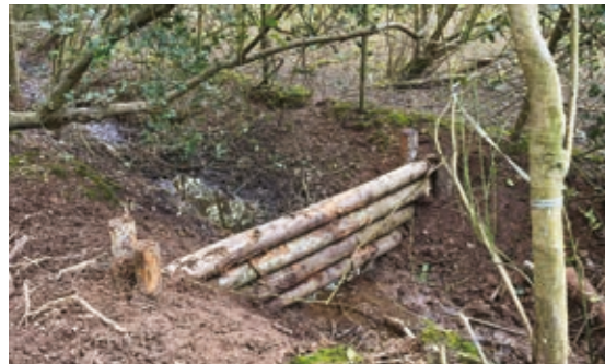
Leaky barrier in Coldharbour Wood
