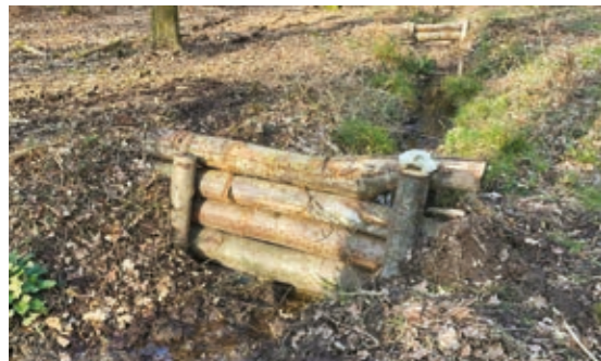
Leaky barrier in St Leger's Copse
