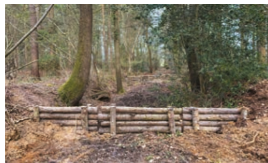
Leaky barriers in Collins Copse
